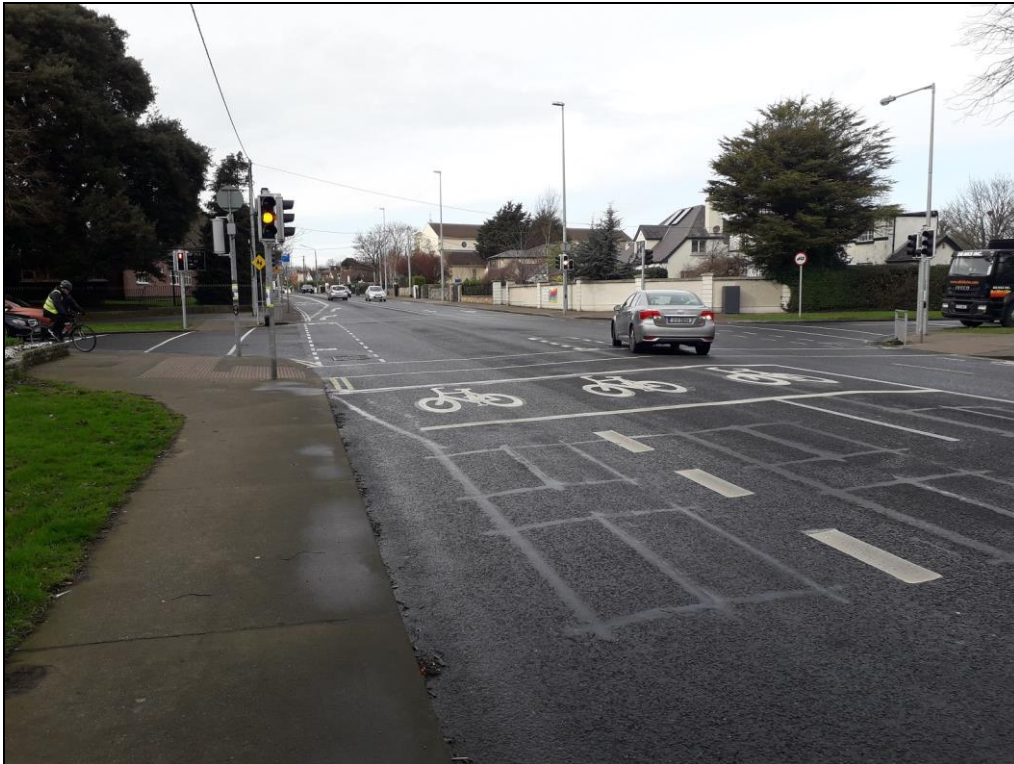
Figure 2.5: Cycle Facilities at Howth Road / Sybil Hill Road junction
